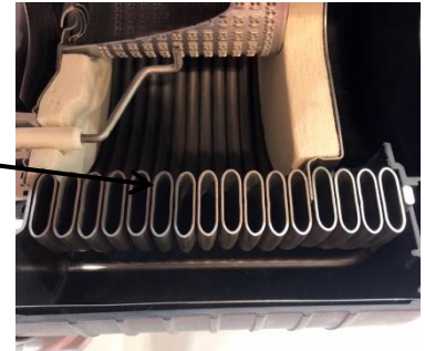
Open Flue Gas Passageways in H.E.
